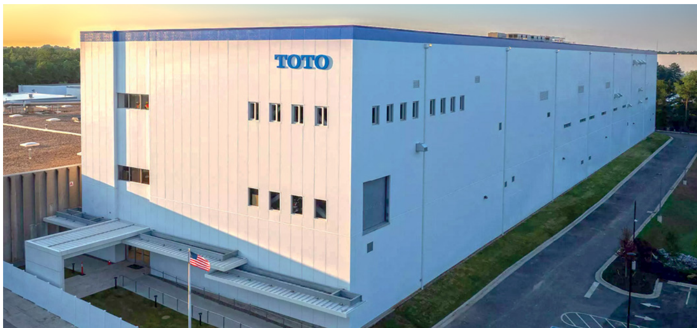
TOTO factory in Morrow, Georgia, USA
